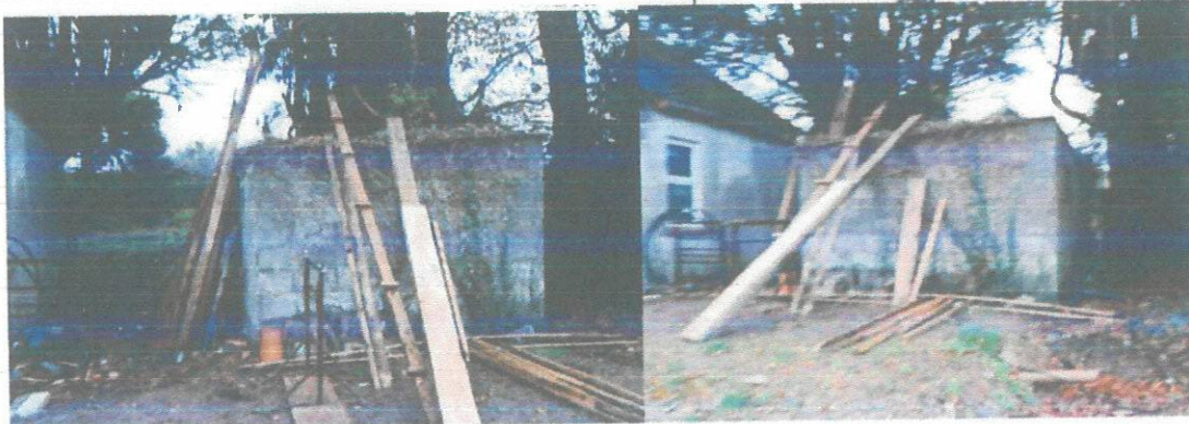
Site inspection 24 th Nov 2021
