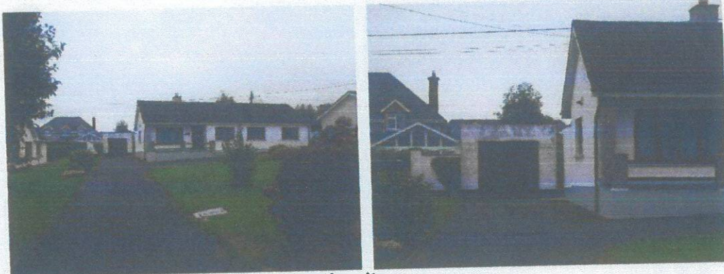
Single storey dwelling and garage on the site
